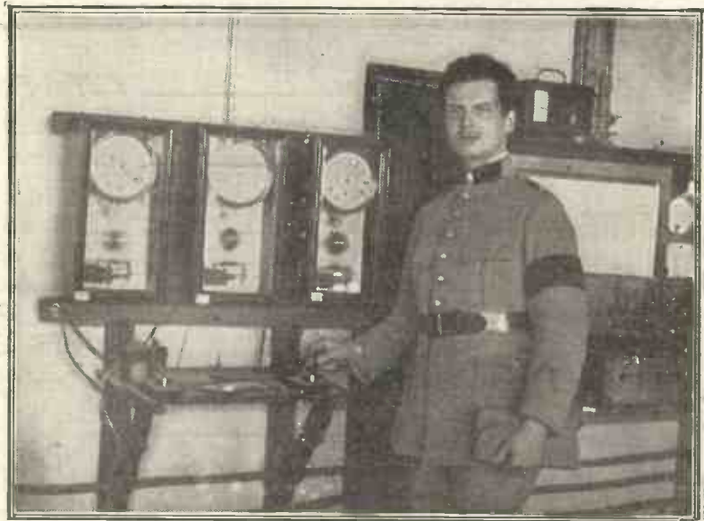
Clocks at the Eiffel Tower station, controlling the time signal emission.
