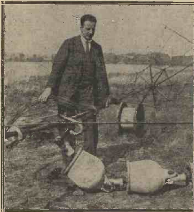
The large objects in the foreground, very much resembling flower pots, will give a good idea of the size of the insulators used in the construction of the giant aerials at Rugby.
