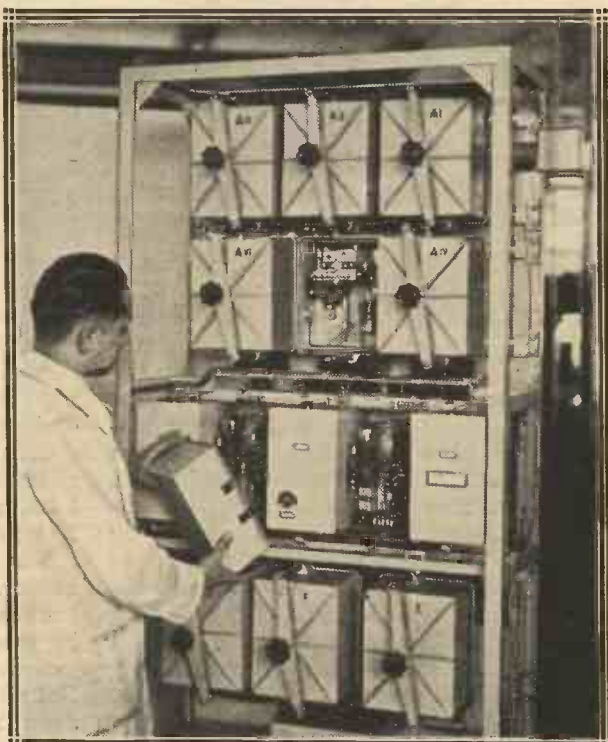
BEHIND THE PANEL of the short-wave receiver used for the Berlin-Tokio telephone service. Beam short-wave transmission and reception is used, the former from Nauen and the latter from Beelitz.
