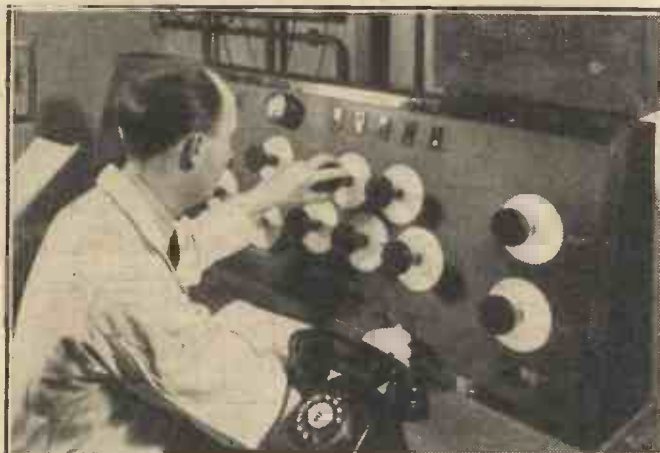
THE SPECIAL CONTROL PANEL in operation. It can mix and balance sound effects, music, and artists recording in eleven different studios for the making of a single record. It cost over £1,000.
