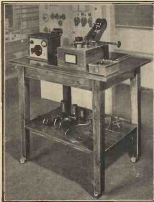
A WAVEMETER used to check up reception on 10-100 metres. The receivers illustrated on the previous page can be seen in the background.
