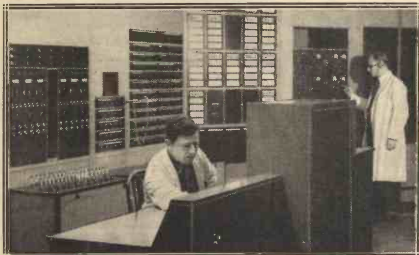
A corner of the control room in Berlin's "Broadcasting House." The indicator in the centre shows which studio is in use and whether for actual broadcasting or rehearsal. The engineer wearing headphones is standing by the checking receivers.
