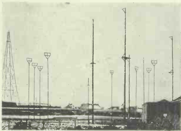
A group of aerials used for the short-wave transmissions from P.C.J., the Philips station in Eindhoven, Holland.
