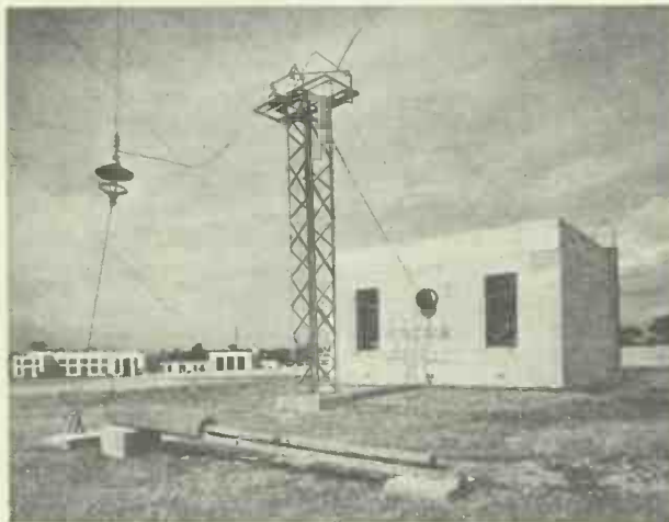
The aerial-transformer house at the B.B.C.'s high-power Droitwich station. The object of P. P. Eckersley's new transmission system is to enable present high-power stations to give better quality, and not necessarily to make room for still more stations.
