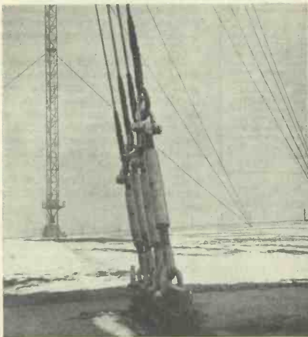
An unusual view of one of the masts at the North Regional station at Moorside Edge. There are three 500-ft. masts supporting the Regional and National aeriels, one mast being common to both aeriels. These aeriels, incidentally, are not of the anti-fading type used at Lisburn. Note the massive anchorages to which the supporting guys are attached. These giant steel masts need very careful staying in order to withstand the severe weather conditions met with in the North.
