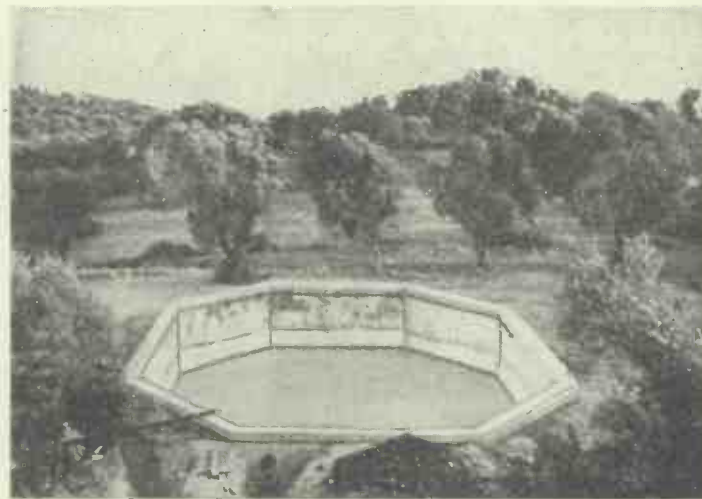
An enormous pond is used to provide the water for cooling the transmitting valves of the new Mediterranean station "Radio-Cote d'Azur."
