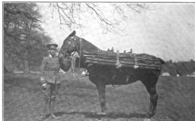
The System Admits of the Masts Being Loaded
