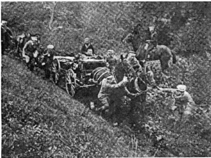
Transporting a Wireless Station over difficult ground.
