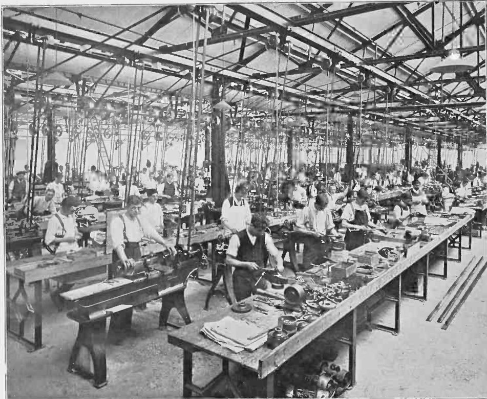
Another View of the Machine Shop.
