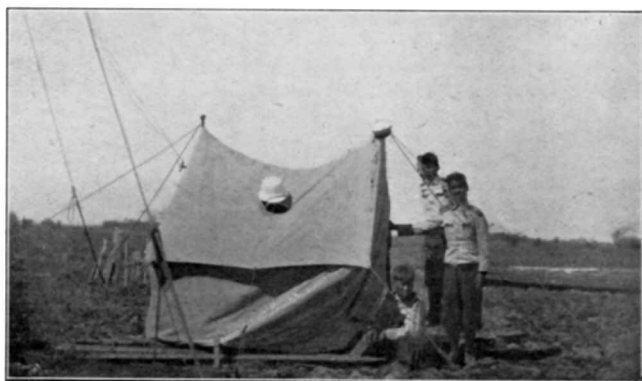
Fig. 8.—A 25 km. Station Operated at Dong Muan during the Manœuvres.
