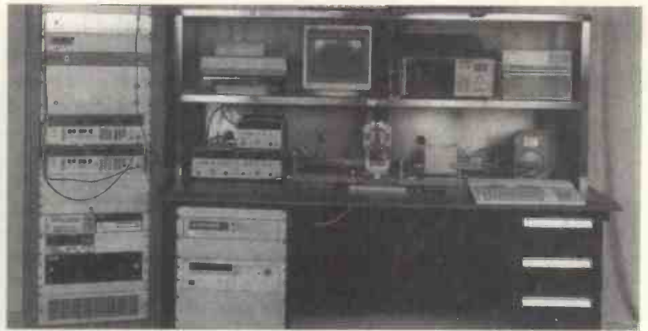
Test station for rf power transistors used by Motorola.
