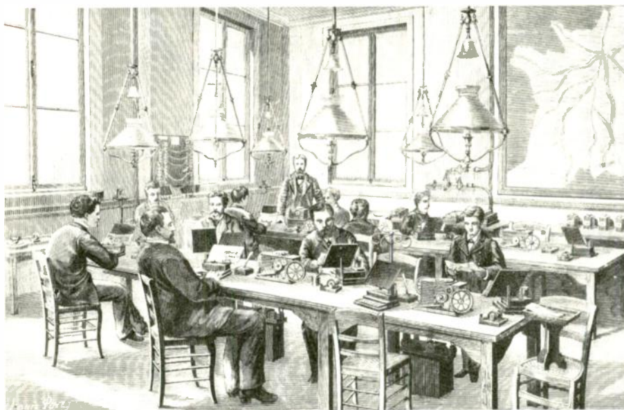
Baudot's multiple printing telegraph, installed at the Administration des Telegraphes in Paris.
