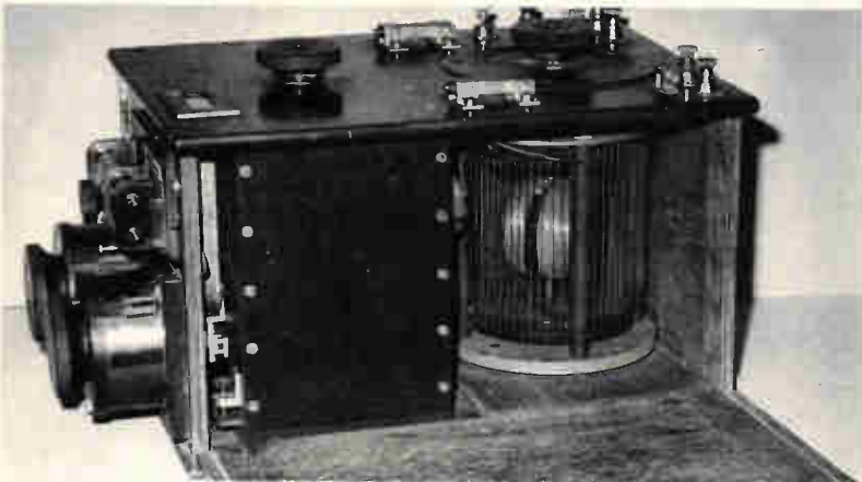
Photo 5. Direction finder of the Marconi-Bellini-Tosi system from circa 1910 helped ships find their position by indicating the directions of known transmitters.
