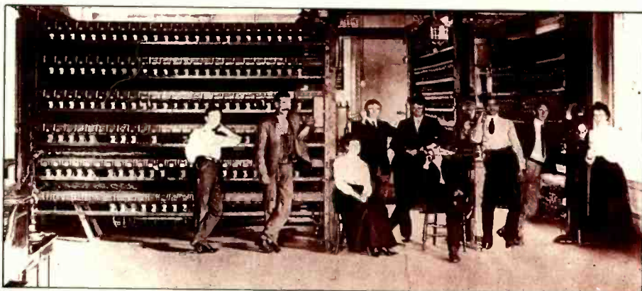
"All things will adjust themselves to the new order": the first Strowger switch installation at LaPorte, Indiana, 1892 (GTE Communications Systems).
