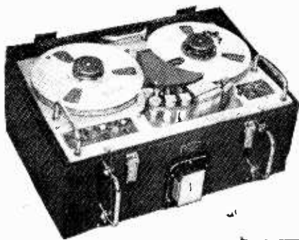
▲ Epsilon MR1080 magnetic recorder for up to 16 channels.
