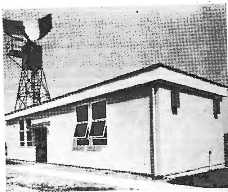
The complete installation. Standard buildings and materials are used, giving a cheap and simple equipment.
