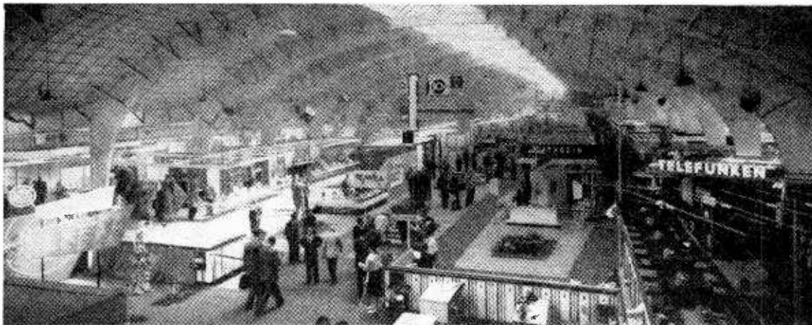
Main hall of the present R.A.I. exhibition buildings in Amsterdam.
