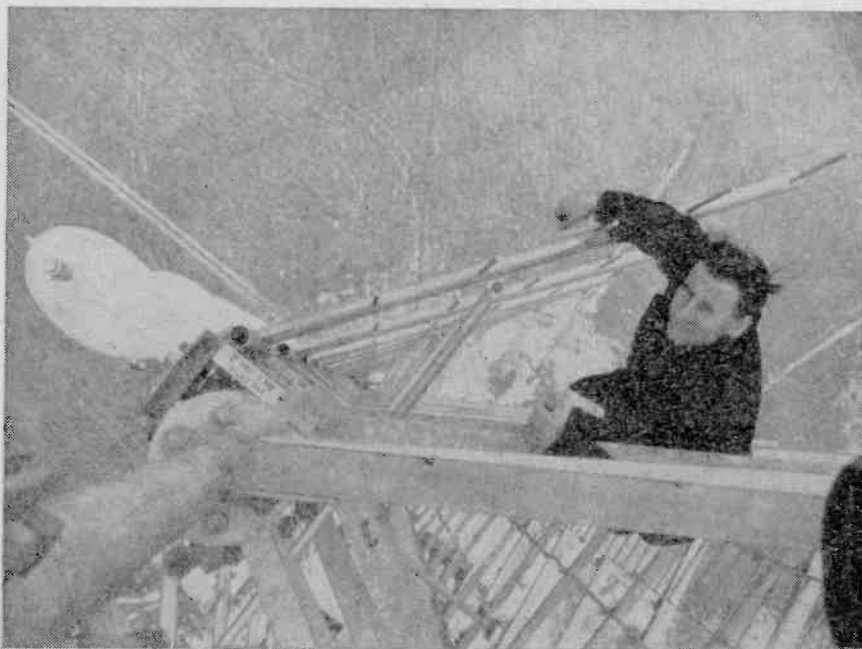
View from above of a part of the dipole structure, showing (left) the anti-icing shields.
