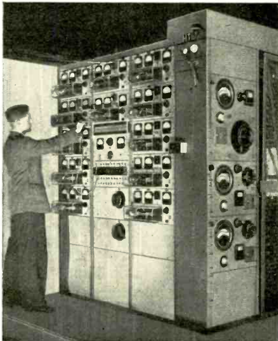
Fig. 5. H.T. enclosure for transmitting-valve life tests.
