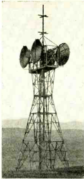
Short aerial tower built into the side of the hill at Blackford Hill, near Edinburgh. The waveguide feeds pass down the centre of the tower.
