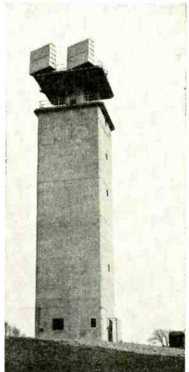
A CHAIN of these concrete towers carrying 10-ft square horn radiators are being erected by the American Telephone and Telegraph Co., to relay television across the States.
