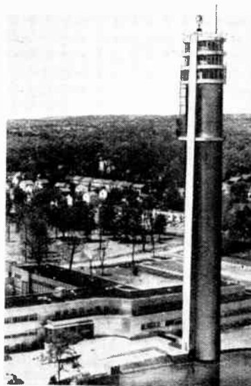
300-FOOT tower recently completed at the Federal Telecommunications Laboratories of the International Telephone and Telegraph Corporation at Nutley, N.J., U.S.A. It will be used for investigating U.S.W. propagation.
