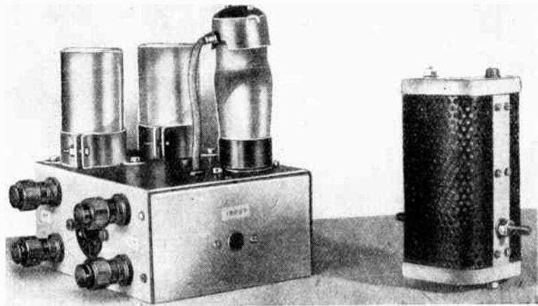
Typical microphone pre-amplifier and (right) experimental ribbon microphone.
