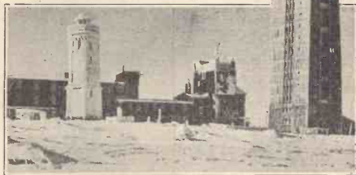
EUROPE'S FIRST mountain-top television transmitter on the Brocken (4,000ft.), which will serve a large area of Central Germany, is housed in the 175-ft. wooden tower on the right.
