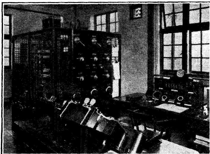
Transmitting and receiving apparatus at North Foreland, the coastal station serving ships bound to or from the Port of London.
