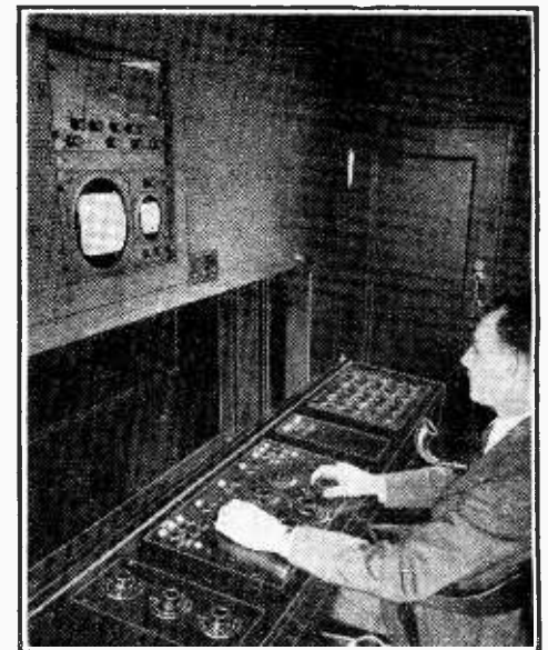
THE VISION MONITOR. Television Control Engineer at the N.B.C. Studio in New York. He controls the outgoing vision transmission and is in direct telephonic communication with the camera operator.
