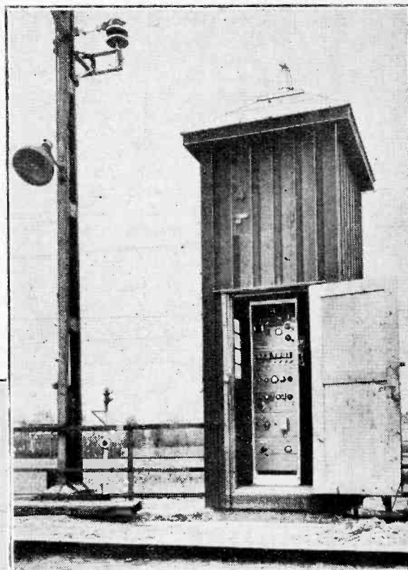
The transmitter is installed in a special housing alongside the track. On the left the shunting official is seen using one of the special control boxes to communicate with the engine-driver.
