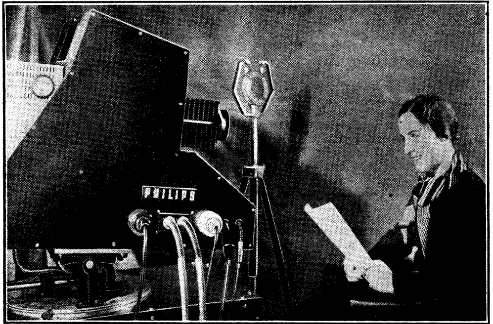
A close-up of the Philips direct television camera.
