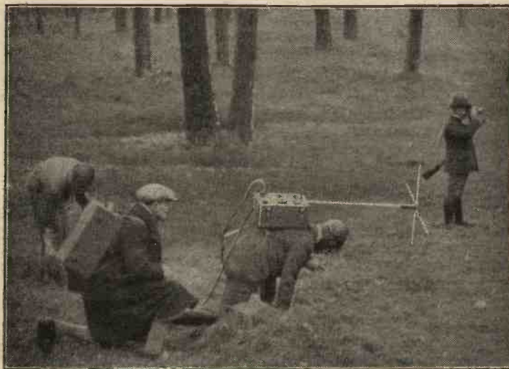
BROADCASTING A STAG HUNT. A Deutschlandssender radio squad at a meet in the former Imperial hunting ground, "Schorfheide," near Berlin. The commentator carries a short-wave transmitter and his companion the batteries. In the rear is the control engineer.
