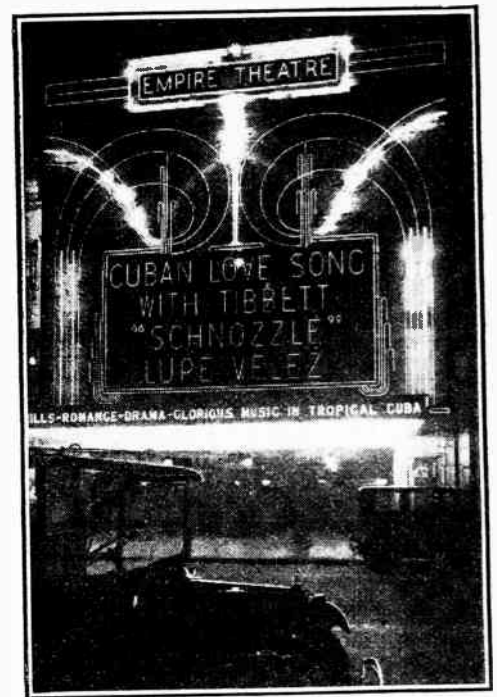
Chokes, condensers and resistances can be brought into use to minimise interference from electric signs.
