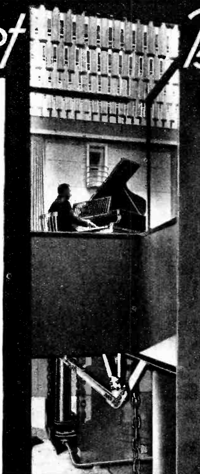
A glimpse of the movable studio floor at Hamburg which can be raised or lowered to vary the acoustic effect.
