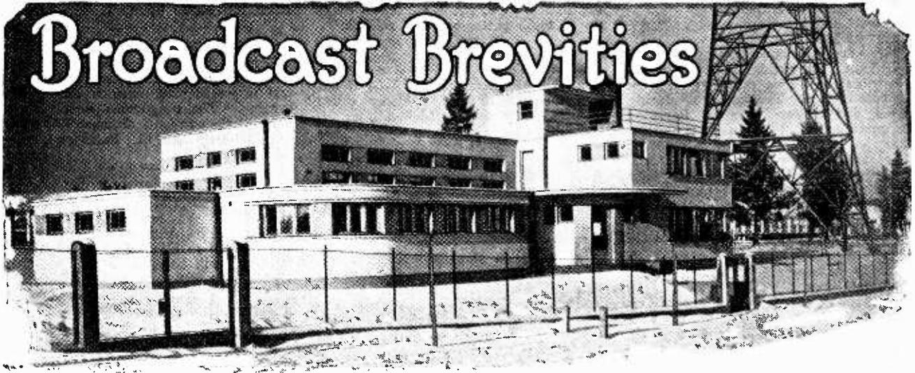
A striking architectural design characterises Lwow (Lemberg) broadcasting station, built by Marconi's for the Polish Broadcasting Company.
