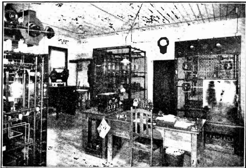
EMPIRE BROADCASTING FROM AUSTRALIA. A recent photograph of the transmitting room at 3LO Melbourne, showing the oscillator, modulator and rectifier panels. The Melbourne station is regularly transmitting a short wave programme on 36 metres every Tuesday between 2.30 and 4.30 a.m. (G.M.T.).
