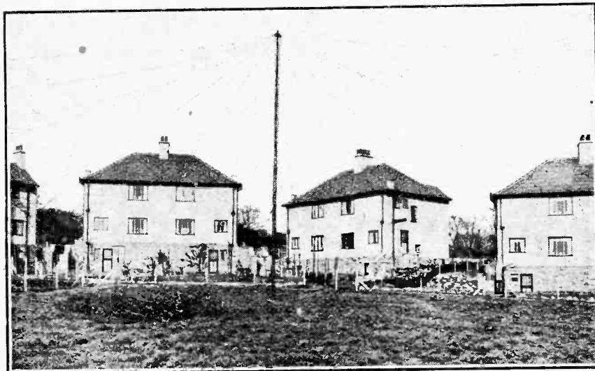
THE COMMUNAL AERIAL. Instead of the usual array of unsightly aerial poles, these new houses of a Bradford estate are provided with the modern "maypole," shown in the photograph.
