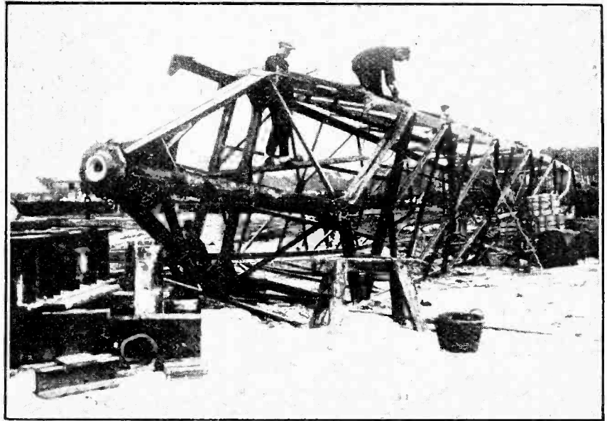
A CALAMITY IN GERMANY. An aerial mast at Königswusterhausen, erected only a few months ago, which has been blown down in a gale.
