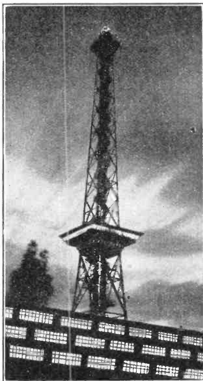
NIGHT LIGHTS. An unusual picture of the new "Radio Tower" of the Berlin Broadcasting Station. A restaurant has been built 200 feet up the 430 feet mast, which is served by a lift that travels up to an observation gallery at the top.
