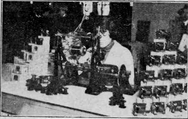
Demonstration of the winding process adopted in the manufacture of Energo transformers.
