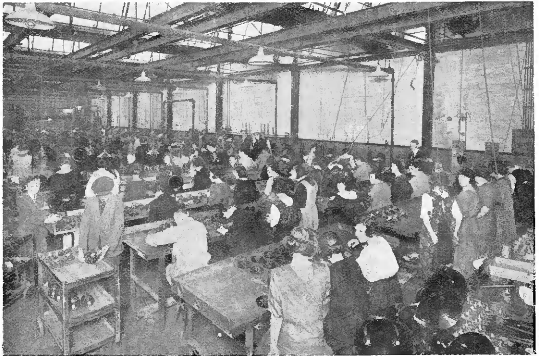
Assembling loud-speakers from finished components.
