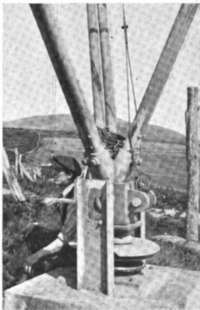
The base of a mast.
