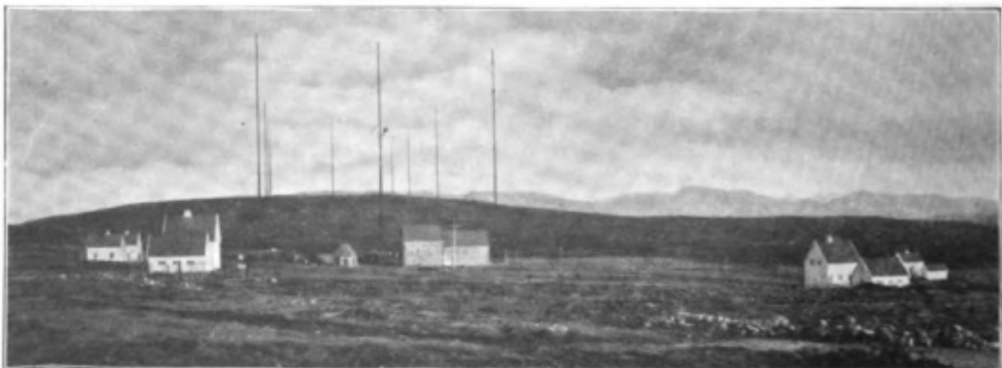
A VIEW OF THE MASTS AND BUILDINGS AT STAVANGER.
