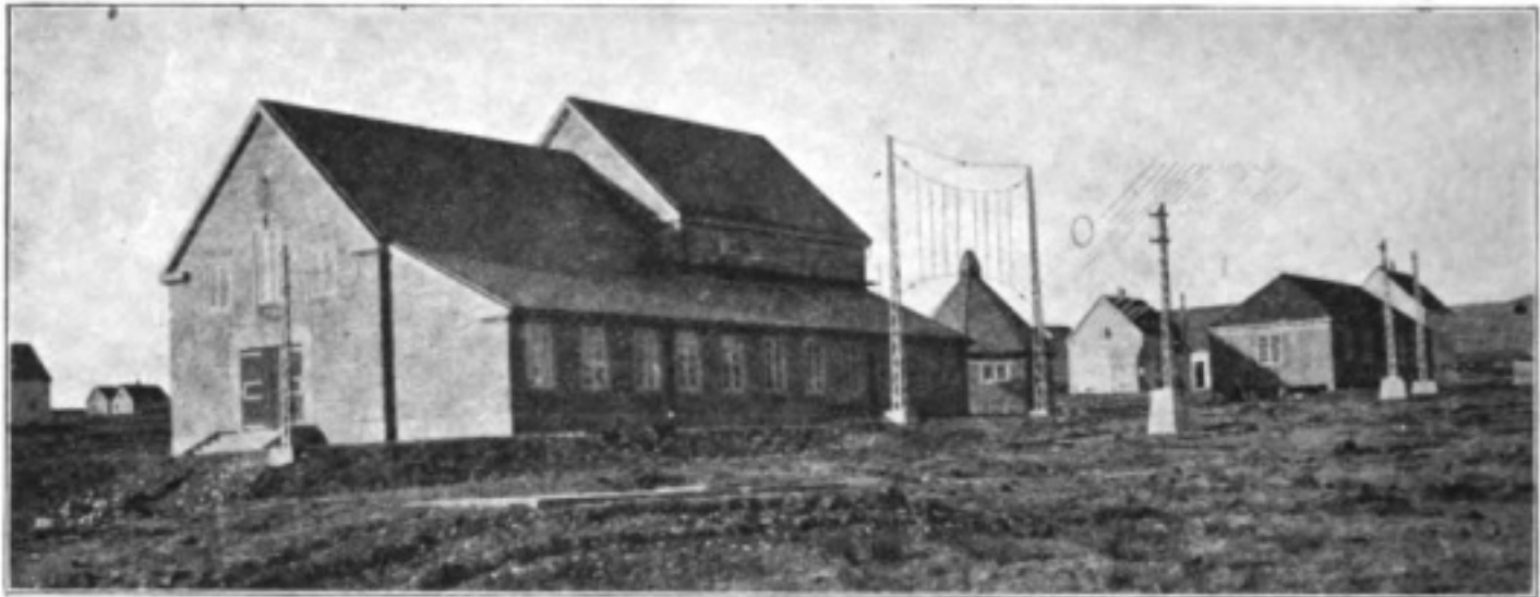
THE TRANSMITTER HOUSE AT STAVANGER, SHOWING THE AERIAL LEAD-IN.
