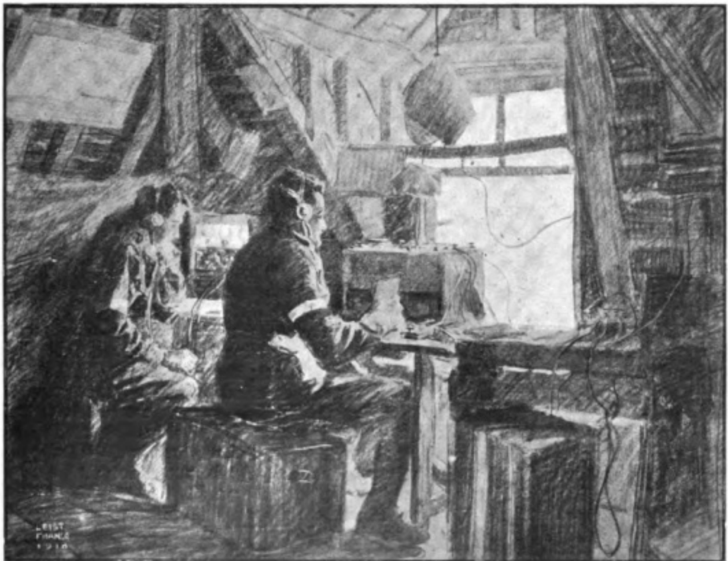
WIRELESS INSTALLATION IN A LOFT ON THE WESTERN FRONT.
