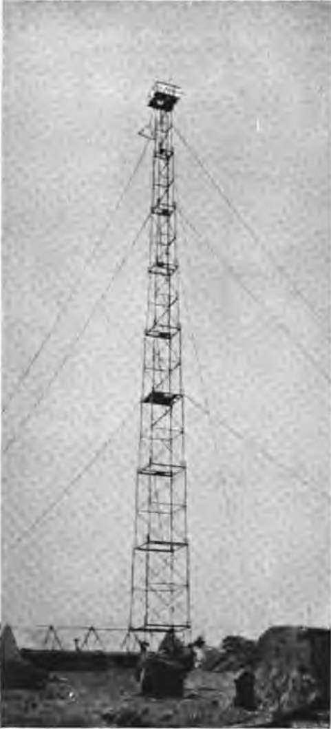
Wireless Tower, Mazatlan.
