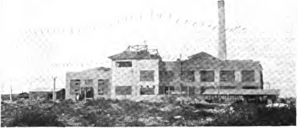
Power House (note Insulators on 32 Aerial Wires).
