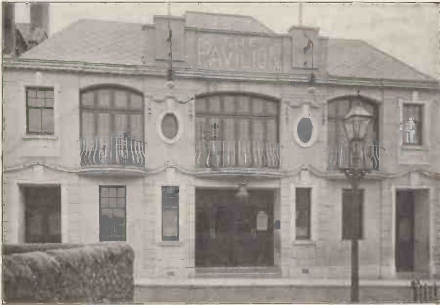
Carnoustie Public Hall White Portland Cement Finish.
