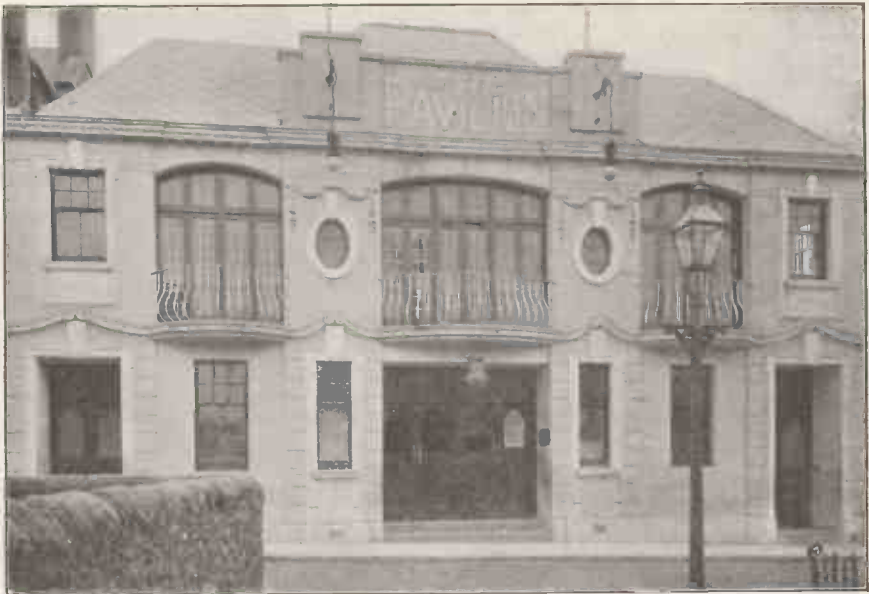
Carnoustie Public Hall. White Portland Cement Finish
