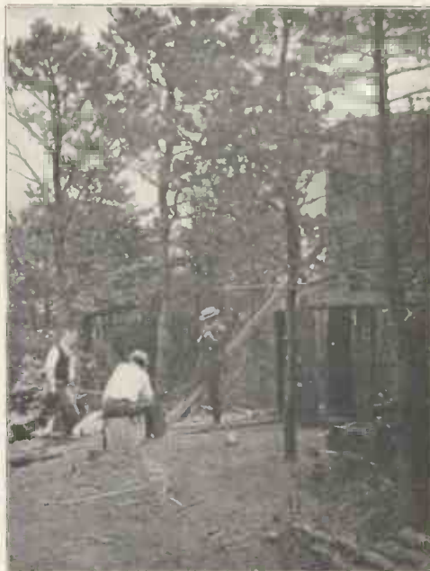
Temporary Water Supply, Chatham Station.
