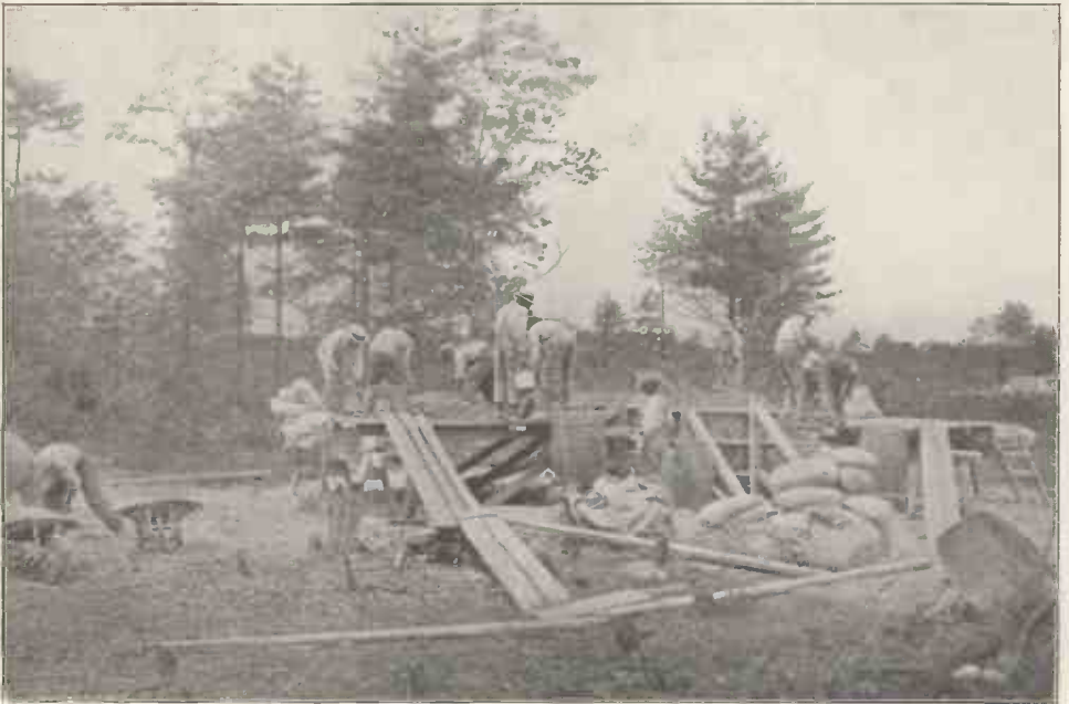
Laying the Foundations of an Aerial.
