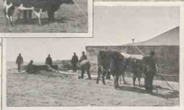
USING OXEN TO MOVE ENGINE FLYWHEEL.
