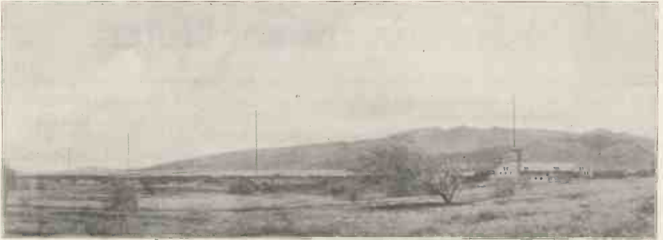
A Panorama of the Marconi Station at Honolulu, showing Power
