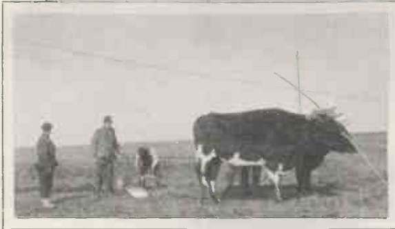
PLOUGHING IN EARTH WIRES.
