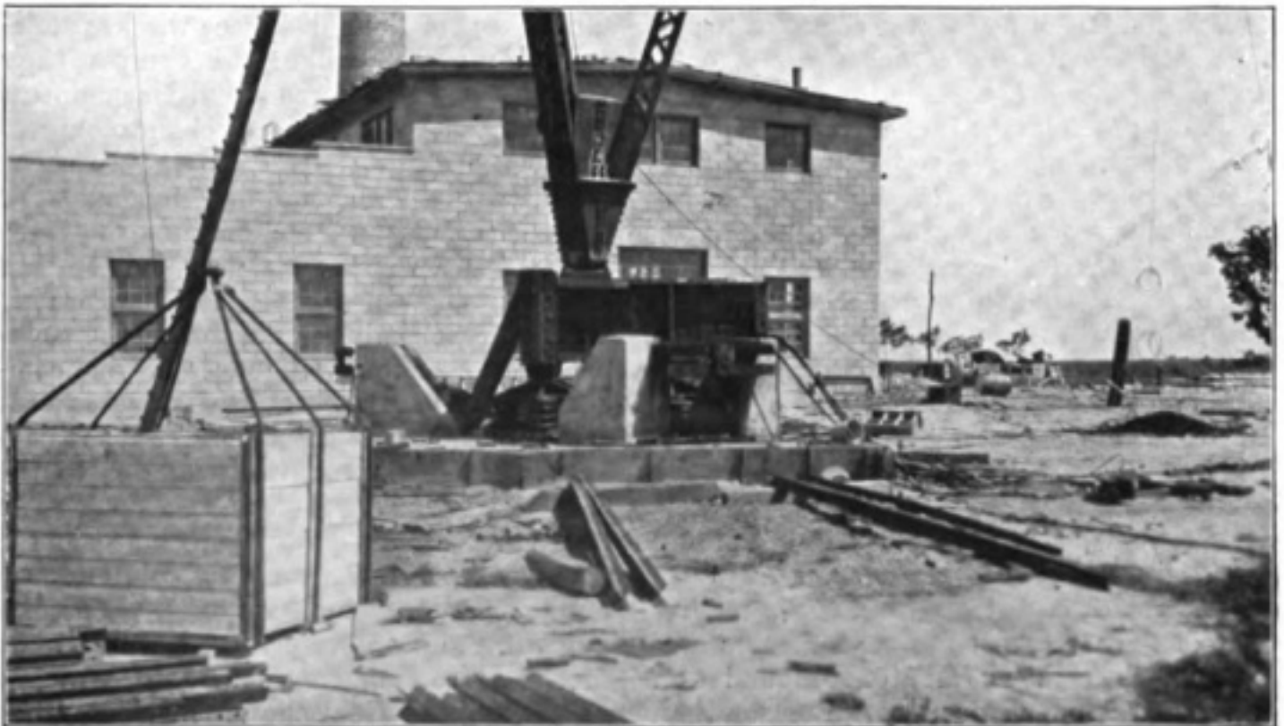
Tuckerton Station, showing the foot of the Steel Tower.
