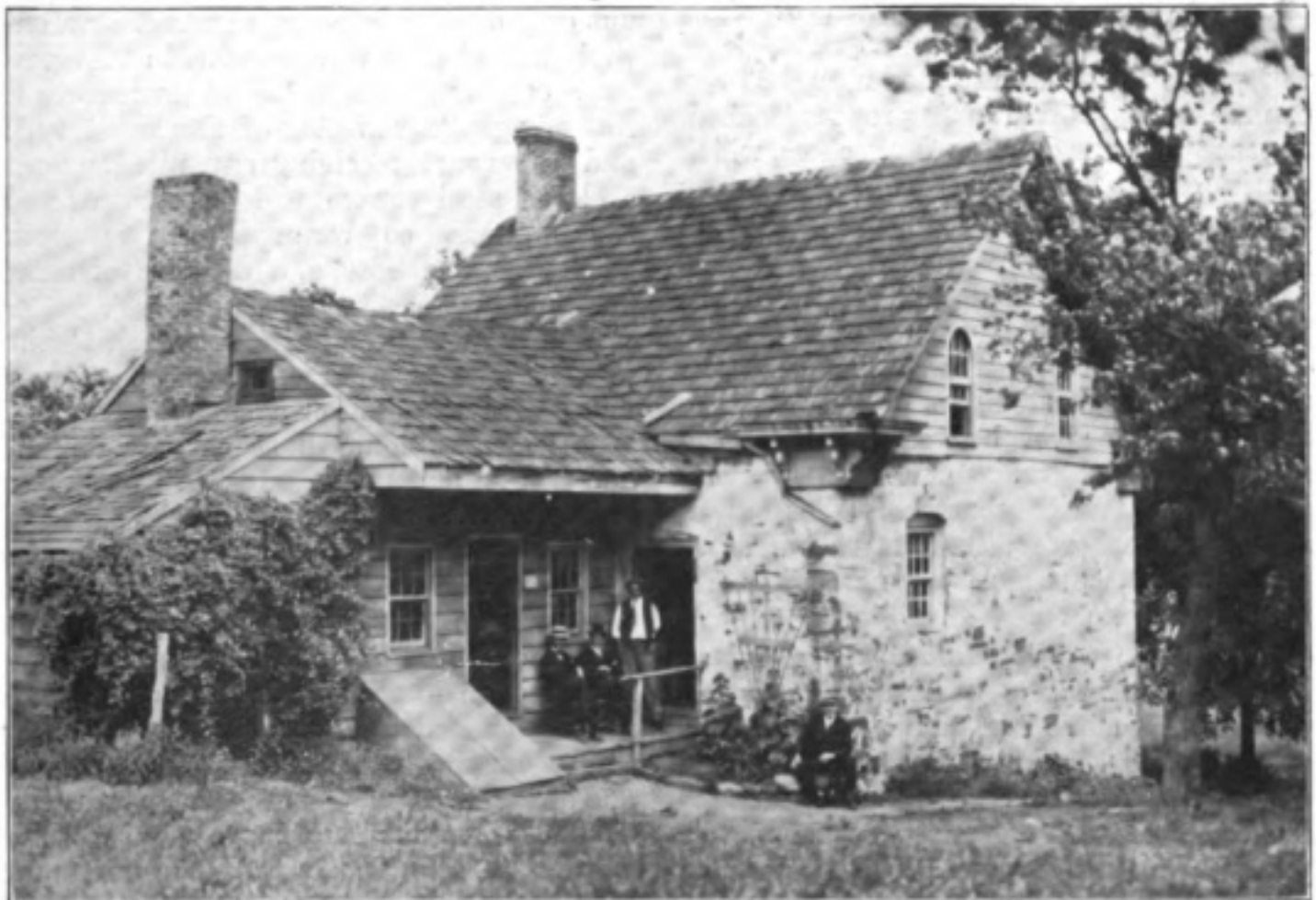
"Lafayette House." An historic dwelling converted to the use of the Staff erecting the New Brunswick Station.
