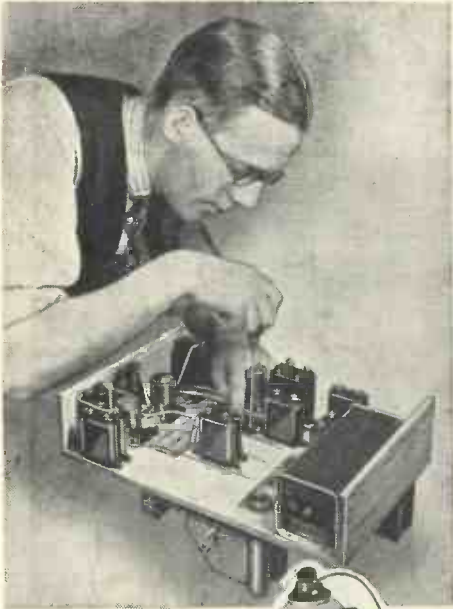
ON WITH THE JOB Here is one of the members of the constructional staff at work on the original set. Note the metal rectifier on the side
