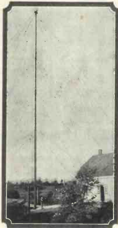
Mast and aerial of the Fyllingen receiving station
