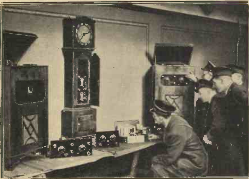
Some of the home-constructed receivers which were exhibited at the annual show of the Nottingham Corporation Transport Radio Club. Among them may be spotted famous S.T. designs, and both an A.C. S.T.400 and a battery S.T.400 won first prizes.
