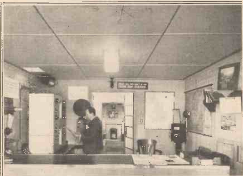
The radio-telephone transmitter at Heston is used for broadcasting accurate weather reports, every hour, for the benefit of the pilots of radio-equipped 'planes. It has a range of about 200 miles and operates on 833 metres.
