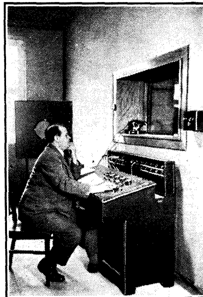
This picture, which was taken in the "Broadcasting House" of the German State Broadcasting Co., shows the panel where music, speech and noises from different studios can be blended before transmission. It provides a striking comparison with the rows of metal-panelled control units favoured by the B.B.C.
